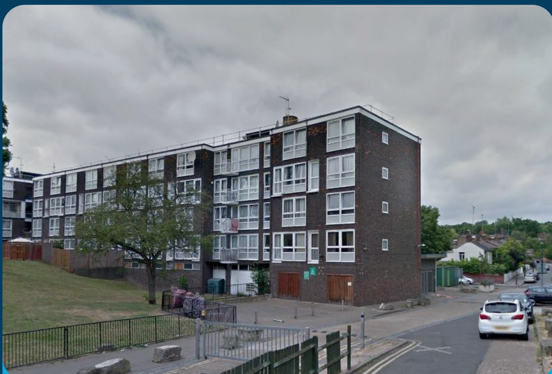
Kiln Place Before
