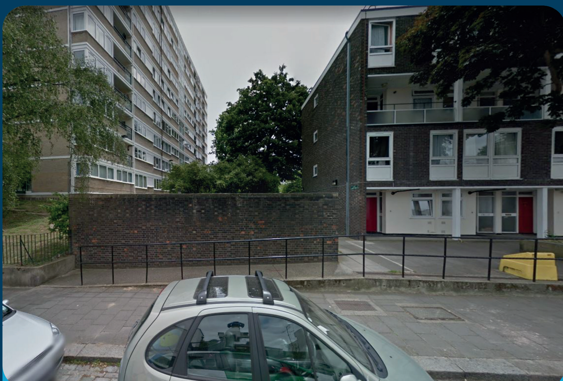
Barrington Close Before
